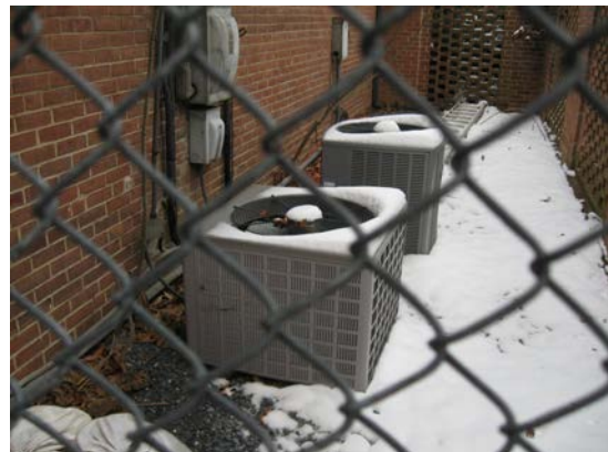
Condensing Units serving AHU-1
